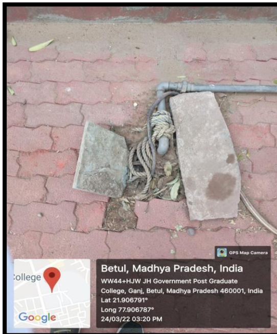
Behind Control Room (Built in 04/03/1997)
