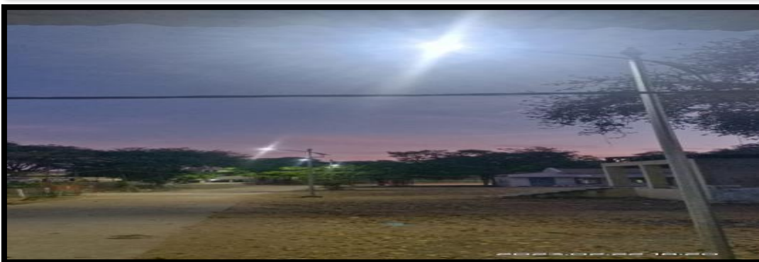
Street lights in College Campus
